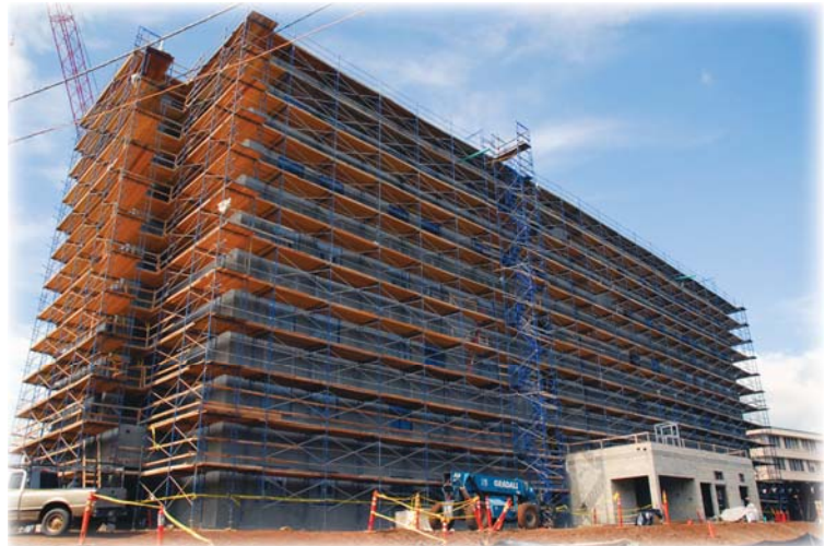
The new Fort Shafter barracks takes shape on Favreau Field, July 2009.
