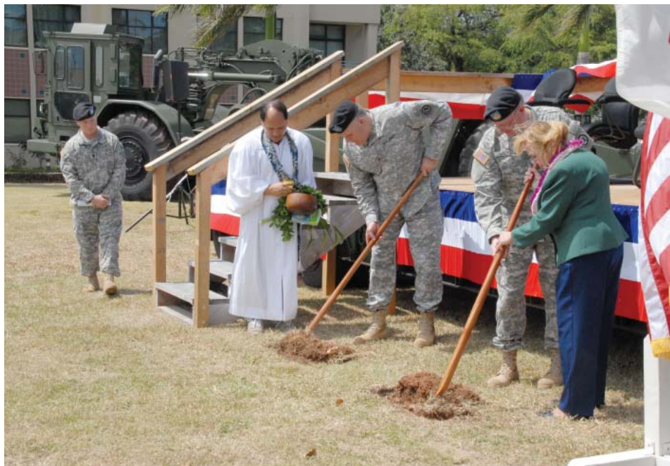
Brig. Gen. Alexander Kozlov (center), outgoing commander of the 9th Mission Support Command, uses a Hawaiian O’o stick to turn the ground signifying the start of construction of the new Army Reserve Center and warehouse at Fort Shafter Flats. Also using an O’o stick (at right) are 9th MSC Command Sgt. Maj. Forrest Wacker and Hawaii Army Reserve Ambassador P. Pasha Baker. Photo by Dino W. Buchanan.
