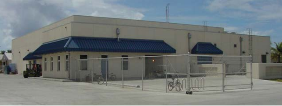
(Left top) A 2007 view of the 150-foot wide ALTAIR and GBP-R (radar) sites on Roi-Namur Island. Courtesy photo (Above) The 22,388 sq. ft. Kwajalein Cold Storage Facility project was completed in 2005 by Dick Pacific Construction Company under a Military Construction Army program. The new facility allows forklifts to drive into the storage rooms thereby greatly reducing man-hours in loading and unloading frozen foods. Photo courtesy of Louis Askew
