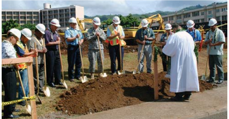
Honolulu District Commander Lt. Col. Jon J. Chytka (center) and construction representatives, project managers and personnel from the Honolulu District, U.S. Army Garrison-Hawaii Directorate of Public Works and project contractor Nan, Inc., bow their heads during the Hawaiian blessing at the groundbreaking ceremonies for the future Favreau Hall. Photo by Dino W. Buchanan
