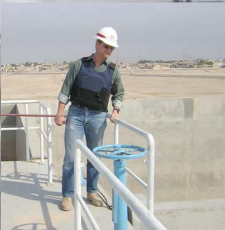
Former Honolulu District civil engineer Bradley Scully checks construction at a water purification plant near Khor Aziz, Iraq during his six-month deployment in 2005.
