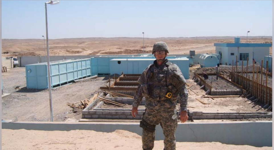
Honolulu District Chief, Real Estate branch Maj. Matthew Luzzatto stands in front a water treatment plant under construction near Kirkuk, Iraq. Courtesy photo
