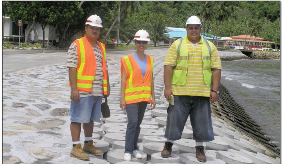
American Samoa Department of Public Works personnel (left to right) Alofa Tanuvasa, construction inspector, Faleosina Voigt, deputy director, Civil Highways Branch and Reuben Siatu'u, project engineer stand on a section of “Samoa Stone” armor units of the $1.4 million Vatia Shoreline Protection project. Courtesy photo.
