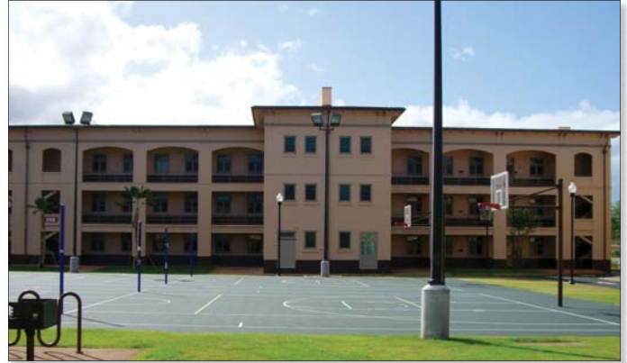
In compliance with Historic Preservation regulations, the Quads remain virtually unchanged while complying with new building codes and anti-terrorism standards. Photo by Frank Ono
