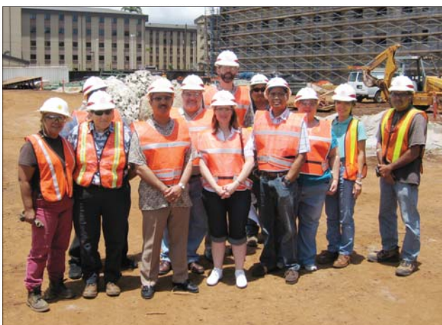
Internal review evaluators from Honolulu, Alaska, Far East, Omaha and Seattle Districts along with employees from Pacific Ocean Division and USACE Headquarters toured the Whole Barracks Renewal Project at Schofield Barracks May 22 to get a clear picture of the district's workload and challenges. The tour was just one facet of the Symposium for IRs organized by Northwest Division's auditor Conrad Gren. Courtesy photo
