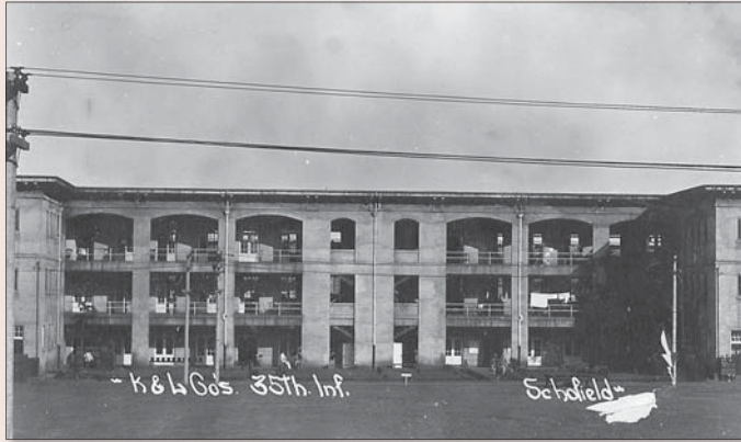
In the early 1900s quad barracks like this one were home to 1,500 Soldiers: one company per floor, with the 1st Sgt. living on one end and the mess hall located on the other. U.S. Army photo
