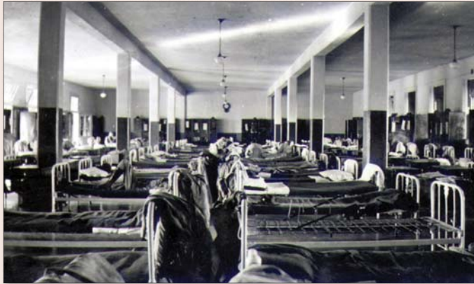
The quads were originally built for "high volume occupancy". Soldiers at Schofield Barracks were issued a bunk and foot locker. U.S. Army photo
