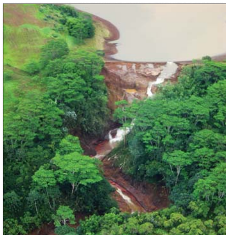
The privately-owned Kaloko Dam (Kauai) breached in March causing the deaths of seven people as millions of gallons of water poured downstream. A PDT was quickly formed to assess the safety of other earthen dams in Hawaii. Courtesy photo
