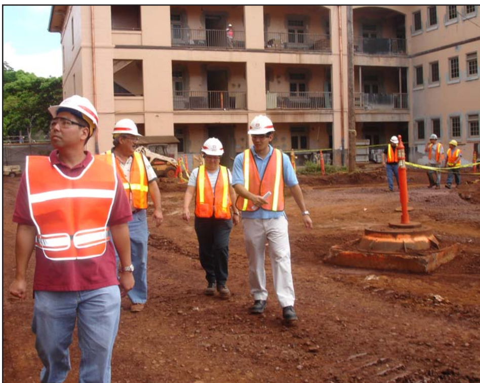
New employee Marc Murashige (left), Frank Ono, Allyn Tabata and new employee Jarrett Hara tour the Quad C renovation project on Schofield Barracks in July. The tour of ongoing projects is just one facet of the POH Overview course which gives new employees the opportunity to see some of Honolulu District's varied missions.
