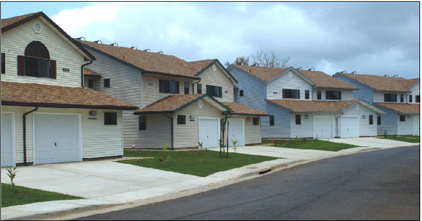
New family housing has been completed at Schofield Barracks for junior non-commissioned officers and company grade officers. The project also includes outside beautification.
