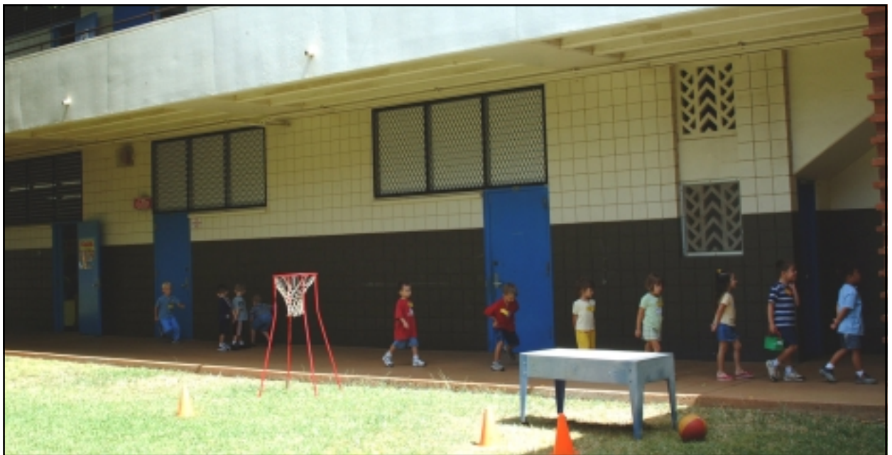
New windows and screens at Nimitz Elementary School provide added ventilation and security.
