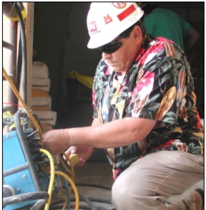
Jeff Cochran, HED’s new safety chief, performs a routine electrical safety check at a job site.
