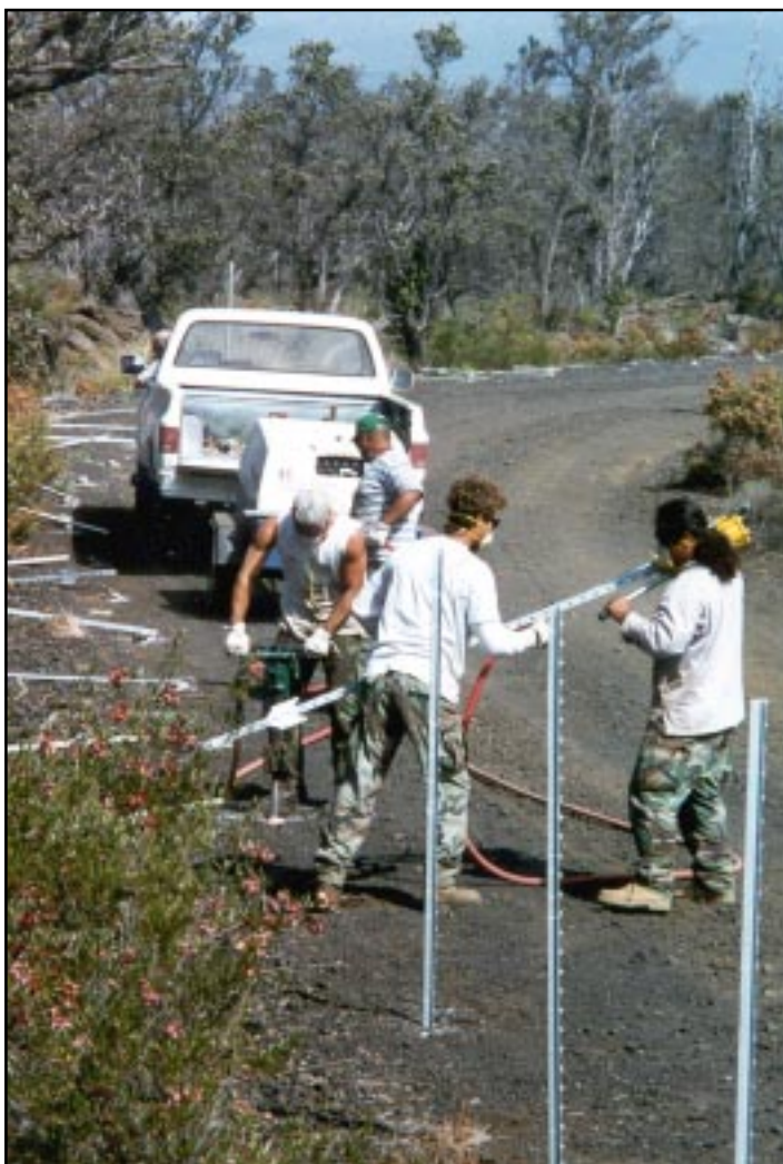
Fence crew installs barrier to protect endangered plants growing close to road within boundaries of Pohakuloa Training Area (PTA).
