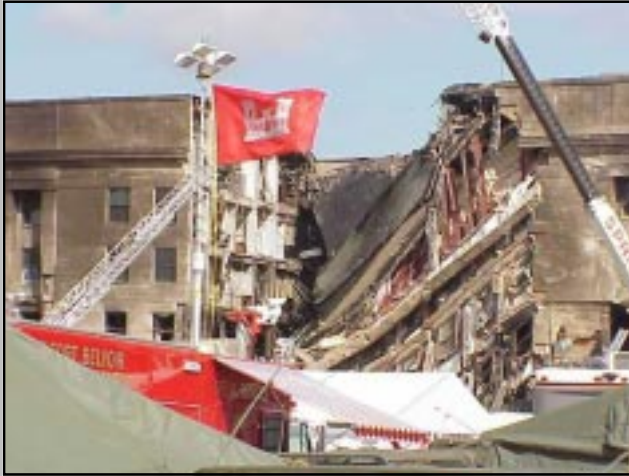
The Military District of Washington Engineer Co. from Fort Belvoir, Va. conducting urban search and rescue operations inside the Pentagon following the Sept. 11 terrorist attack. — U.S. Army photo.
