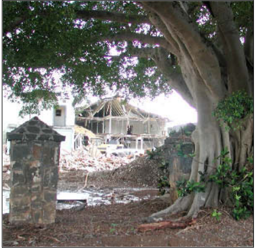
These two stone pillars behind the rapidly disappearing T-1 once marked an entrance to Fort Shafter.
