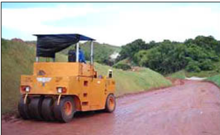
Palau gets as much as 150 inches of rain a year, making soil compaction, a key element of road building, difficult. —Photo by Lt. Col. Ronald Light.
