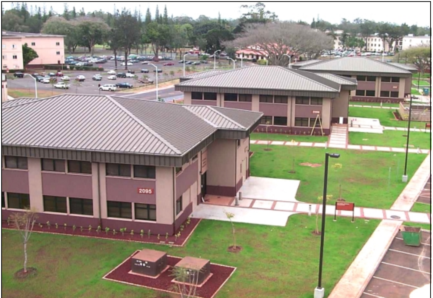
These three battalion headquarters buildings, part of the FY99 contract for Phase I of the Whole Barracks Renewal project going on at Schofield Barracks, are nearly completed and the units from 2nd Brigade, 25th Infantry Division will be able to begin moving into them in March. —Photo by Kimberly Jyo.
