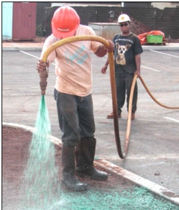
Workers put the final touches on the landscaping of 2nd Brigade, 25th Infantry Division’s new battalion headquarters buildings. —Photo by Michelle Cain.
