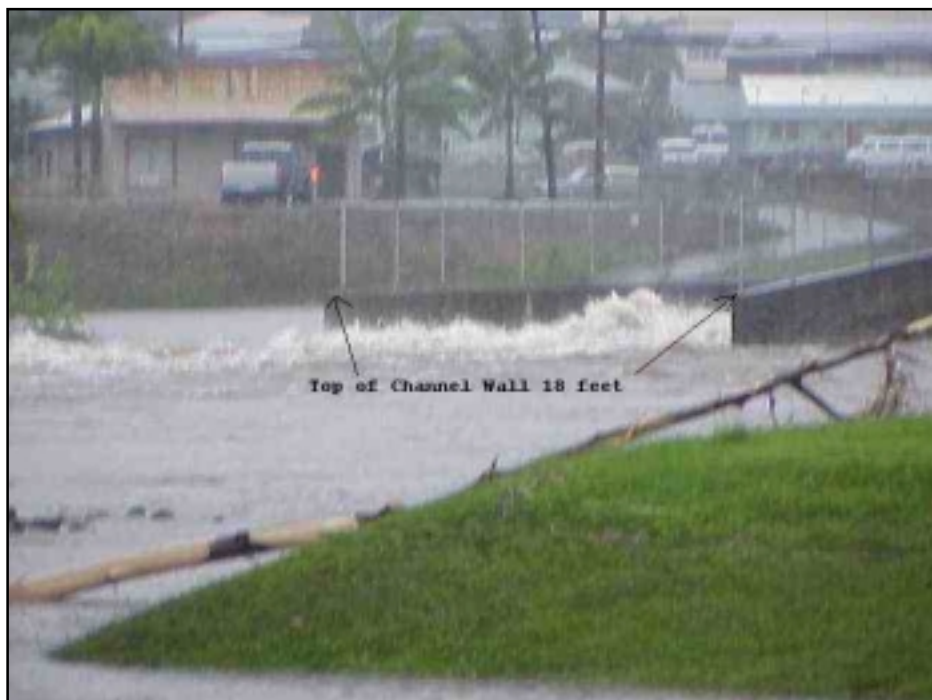
Alenaio Stream outlet showing water level as it exits the flood control project.
