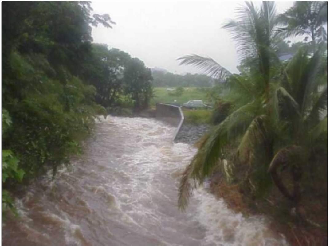
The Alenaio Flood Control Project is functioning near capacity carrying a torrent from 37 inches of rain in two days. —Photo by Dan Meyers.
