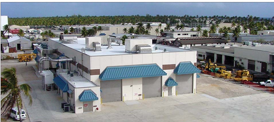
Honolulu District’s Kwajalein Resident Office (KRO) managed the $10 million, 20,000 square foot VPP project which includes rooms for hydro blasting and undercoating, booths for abrasive blasting, metallization and paint spraying. Photo courtesy of USAKA Public Affairs Office
