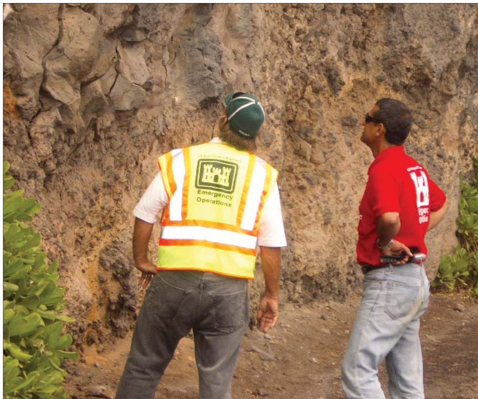
HED Geologist Eric Bjorken and Sacramento District's Ghassem Khosrownia perform a visual inspection for potential hazards caused by the Oct. 15, 2007 earthquake on the island of Hawaii. Courtesy photo
