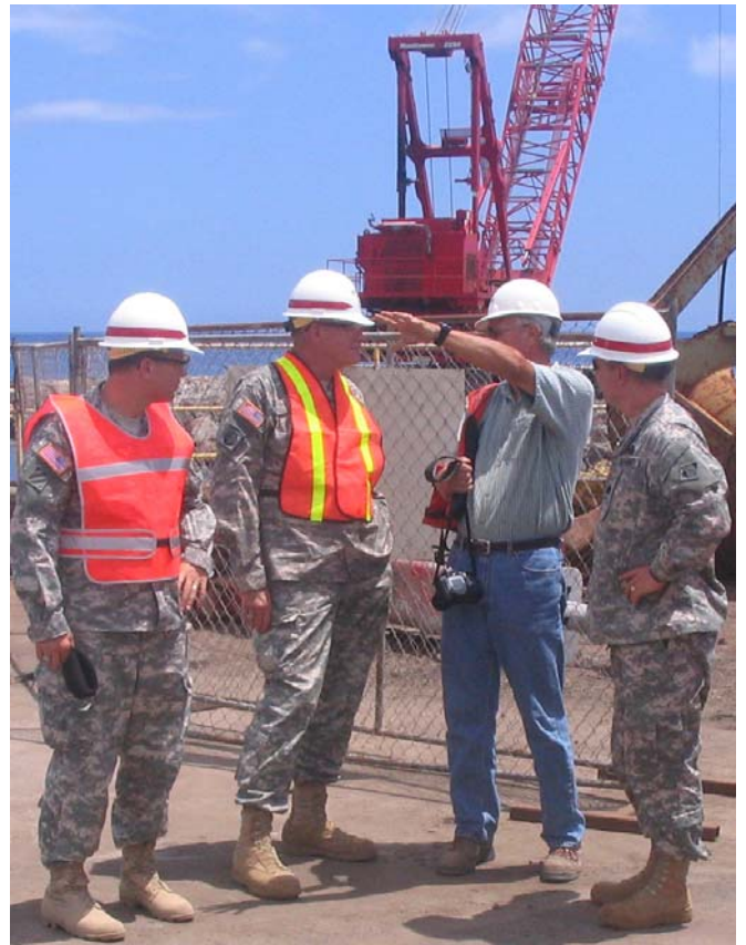
Traylor Brothers (Pacific), Inc. Project Manager John Gustafson explains the Kaunalapau Harbor project to POD Commander Col. John W. Peabody, Chief of Engineers Lt. Gen. Carl A. Strock and Honolulu District Commander David E. Anderson. Photo by Jim Hatashima
