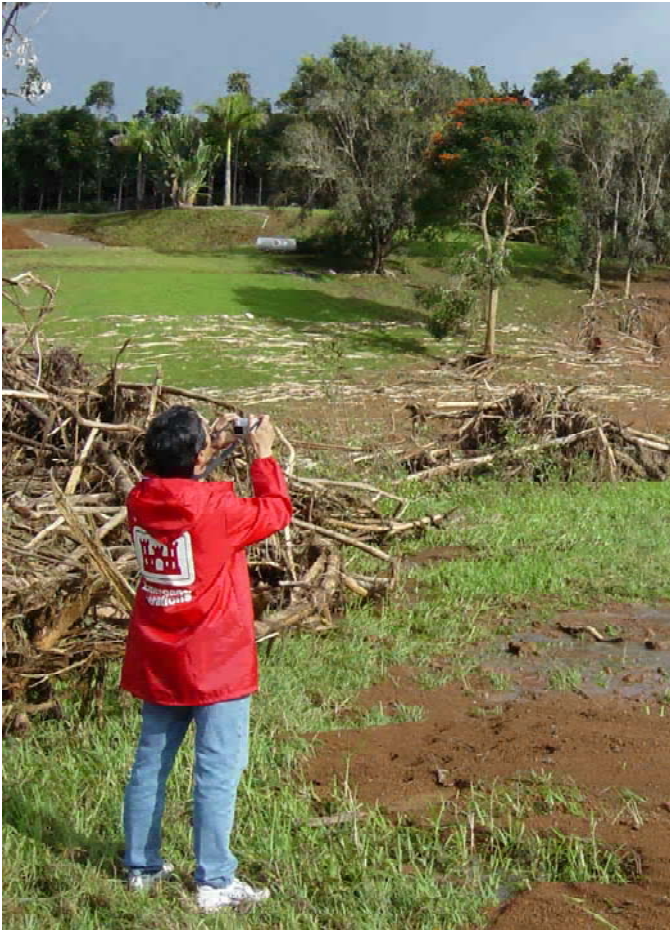
Civil Engineer Ray Kong photographs a Kauai dam site March 15. Honolulu District assisted Hawaii Dept. of Land and Natural Resources with emergency dam inspections after the Kaloko Dam breached on March 14. Photo by Lincoln Gayagas
