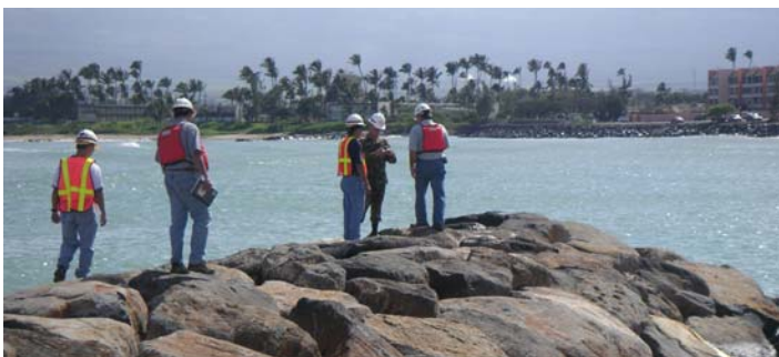
Honolulu District and contractor Healy Tibbitts employees inspect the completed Kahului Light Draft Harbor project in Maui. The $3.6 million DLNR-HED project included deepening and widening the harbor, constructing three boat ramps and a loading dock. Courtesy photo
