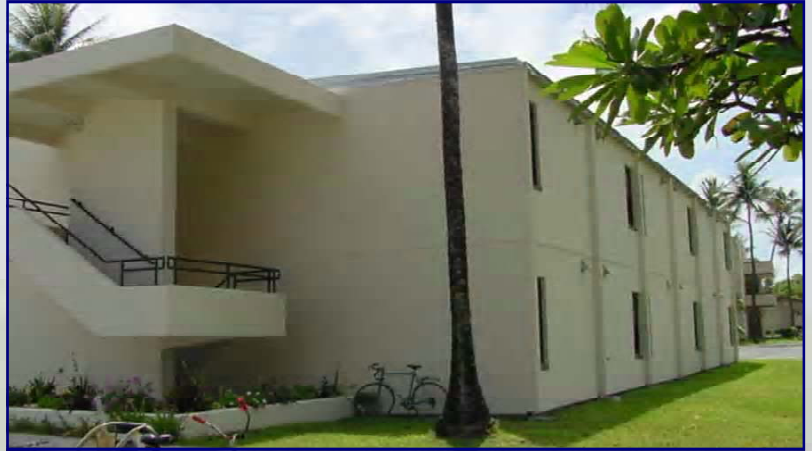
Feb. 7: Single military members move into the newly renovated bachelor quarters in Kwajalein. The $1.8 million project improves the quality of life for Soldiers.
