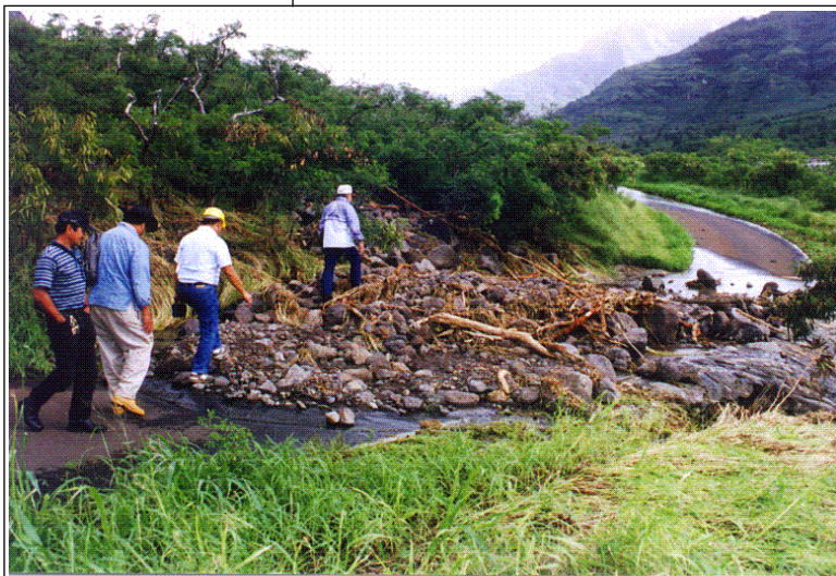
(Top) Checking out damage to the water wells access road in Makaha. (L to R) Gary Morinaga, Honolulu Board of Water Supply; Ronald Ching, Division of Public Works, Hawaii; Clayton Ching, Hawaii Civil Defense System; Harry Aoki, POD ET-TE. (Bottom) Steven Yamamoto, POD ET-PP, rendering assistance to a Nanakuli resident stalled in floodwaters on Paakea Road.
