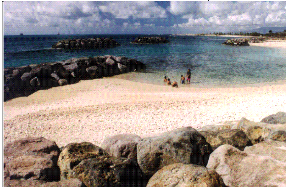
(Below) The Sand Island State Park shore protection project, a joint venture between the state of Hawaii and the U.S. Army Corps of Engineers, Honolulu District. Completed and dedicated in October, 1991, the revetment (bottom center) now protects the park's westward coastline and complements the park with a newly created beach and wading pool together with walkways and landscaping. The pre-project photo (bottom right) shows the extreme soil erosion caused by constant wave action.
