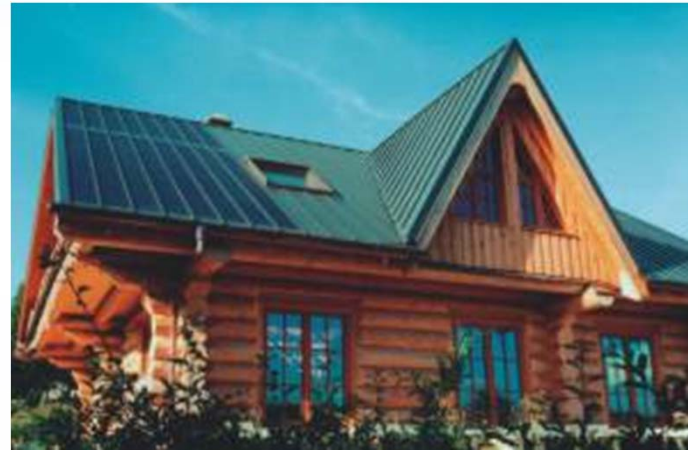
3kW a-Si rooftop at Sandia's Distributed Energy Technologies Laboratory (DETL)
