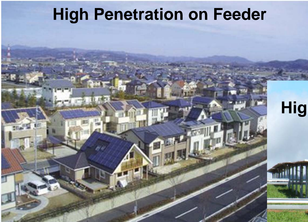
Ota City, Japan: 2 MW PV on single feeder (553 homes, 3.85 kW average PV system)
