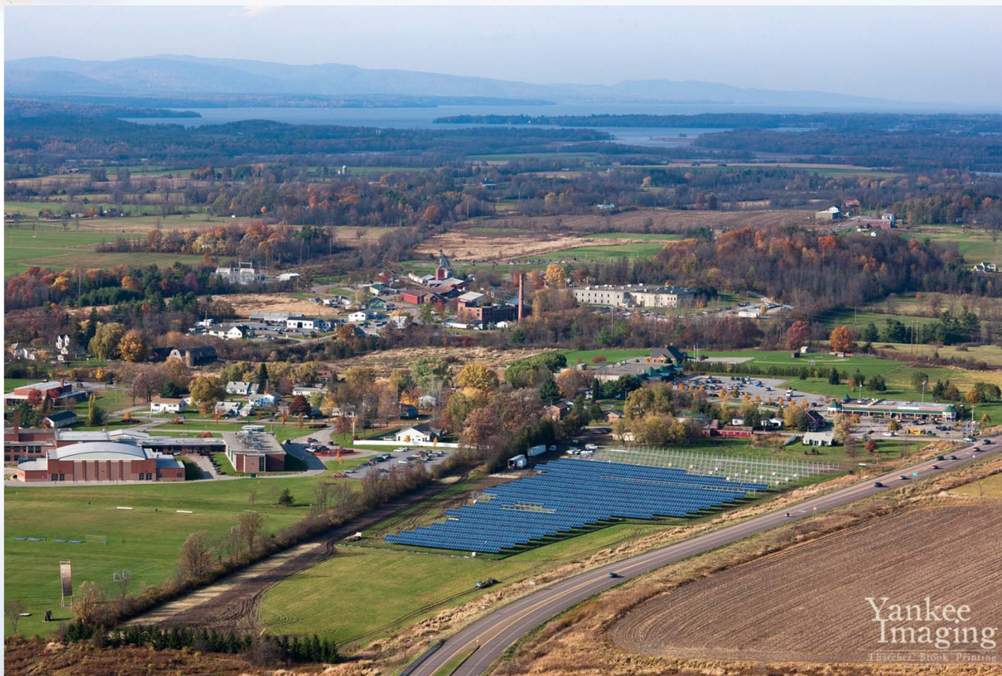
Ferrisburgh Solar Farm, Vermont
