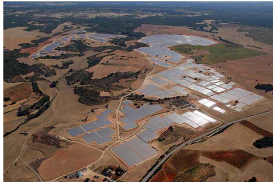
Olmedilla Park Solar Power Plant (60 MW)
