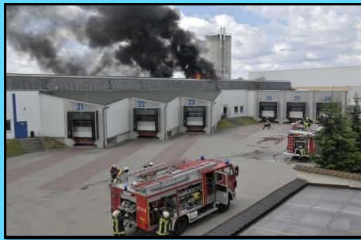
PV arc fault-initiated fire on a warehouse in Buerstadt, Germany.
