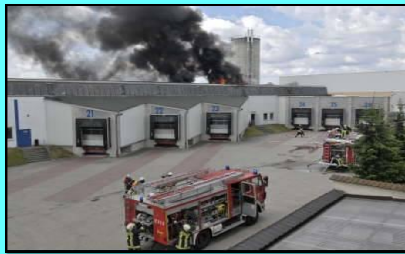
PV arc fault-initiated fire on a warehouse in Buerstadt Germany.
