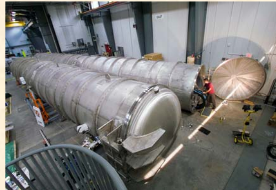
Installation of SANS instruments
