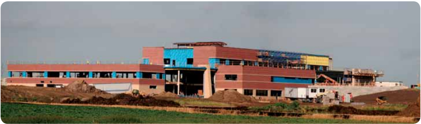
Jamestown Regional Medical Center under construction.
