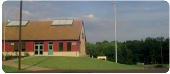
New solar panels and a wind turbine help Salem Children’s Trust conserve energy and cut costs.
