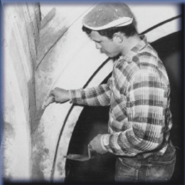
CO patching a wall in a school damaged during World War II in Vienna.
