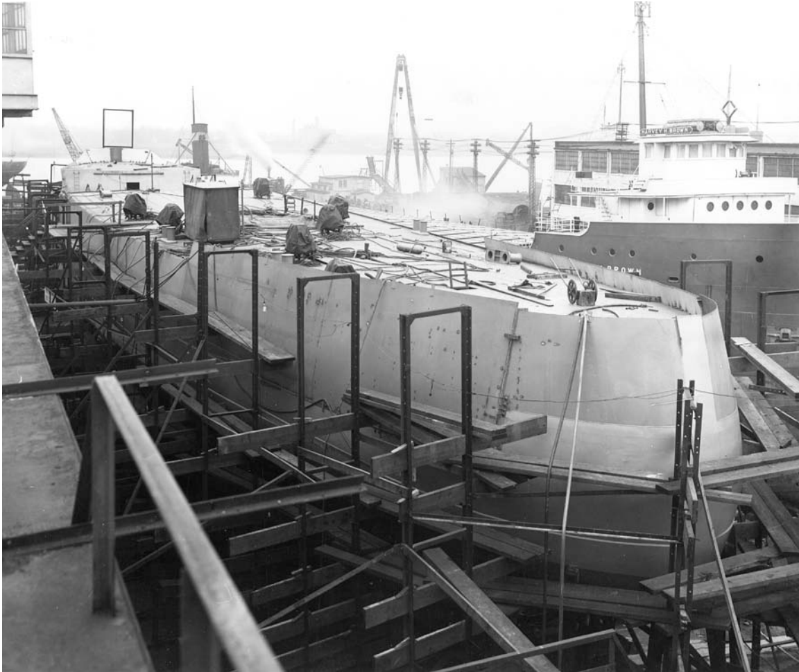
Storis under construction, 15 March 1942.
