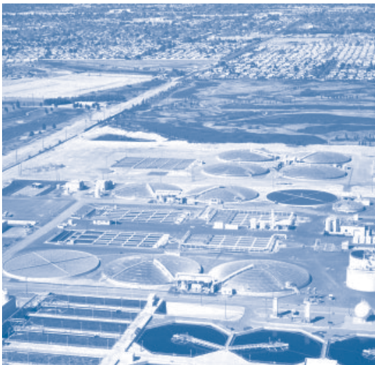
Wastewater treatment plant Source: Natural Resources Conservation Service
