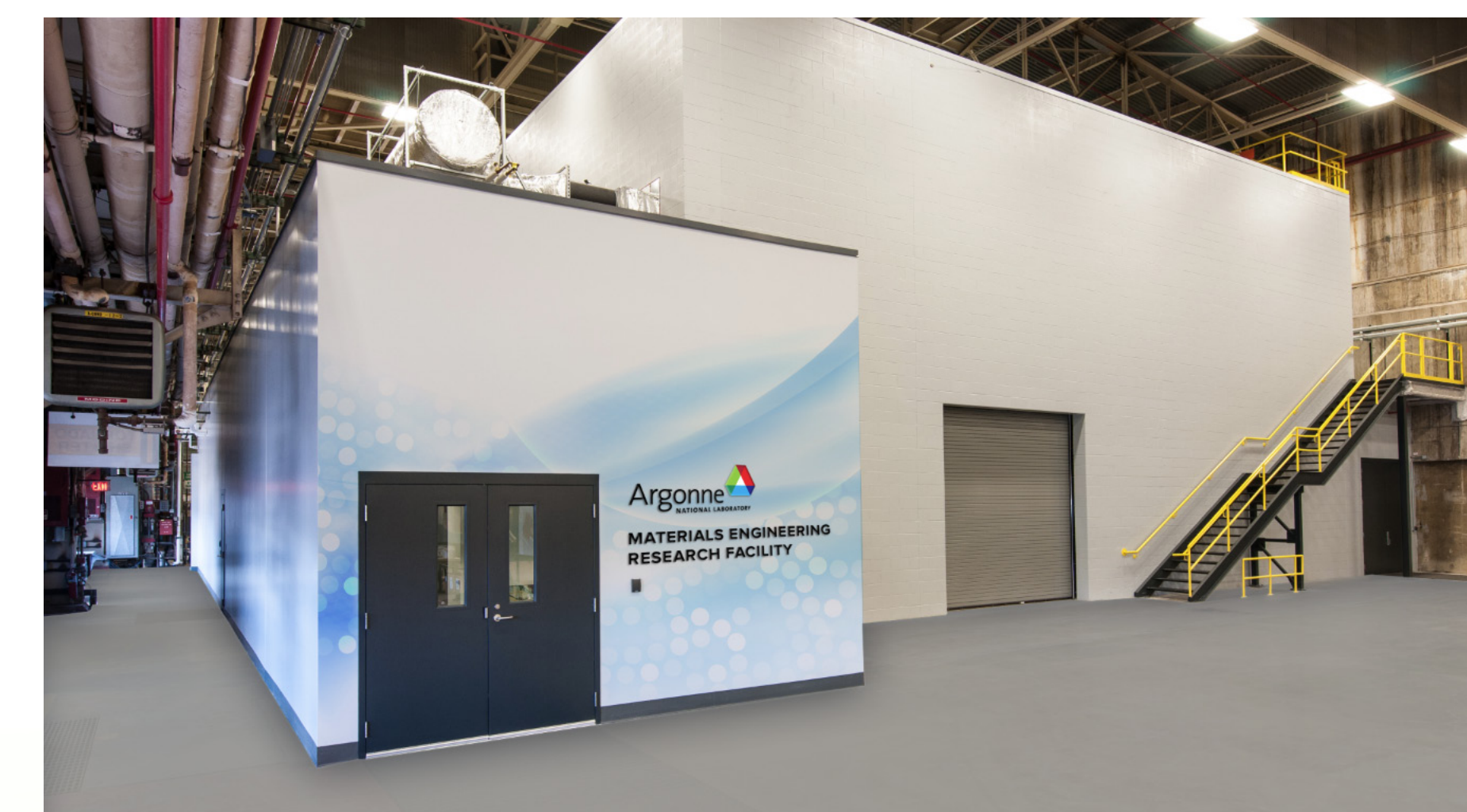
Argonne's Materials Engineering Research Facility.
