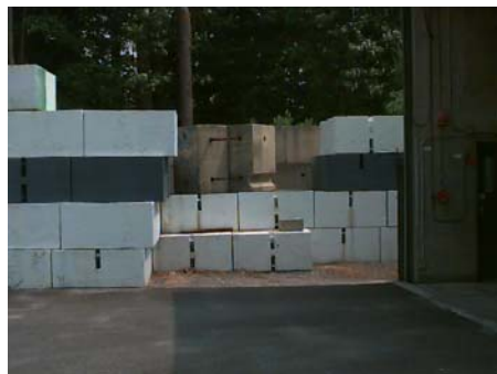
Shielding Blocks at the Hall C Truck Ramp Entrance
