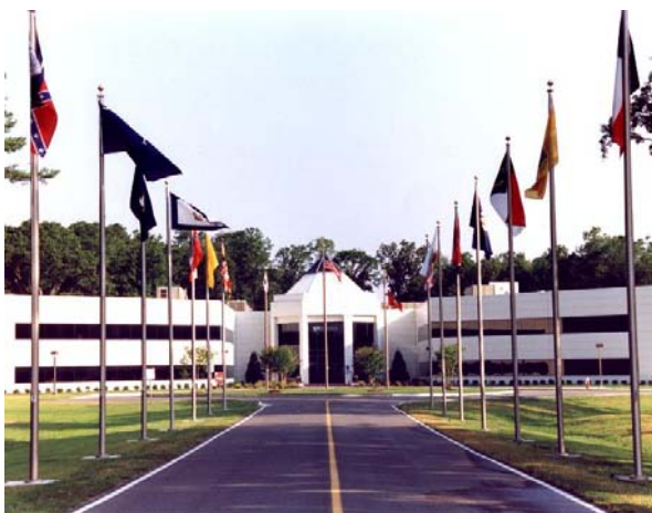
Front Entrance to CEBAF Center
