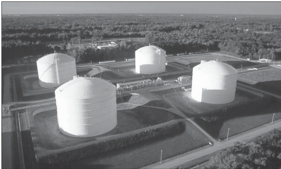
Dominion's Cove Point liquefied natural gas import facility on the Chesapeake Bay in Cove Point, Maryland. © 2002 Cameron Davidson
