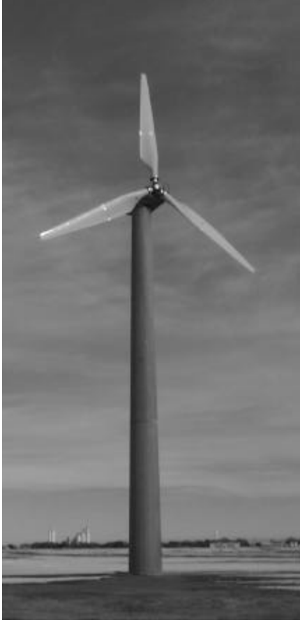
Fig. 1. The Micon 65/13M turbine at the Bushland Test Site.
