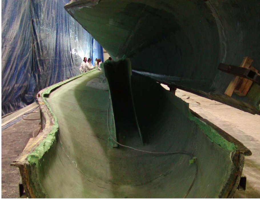
Figure 4.11 Bond assembly of the KC-51 blade at Knight & Carver in San Diego.
