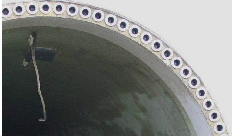
Figure 3.9 Vestas V80 blade with bonded threaded inserts.
