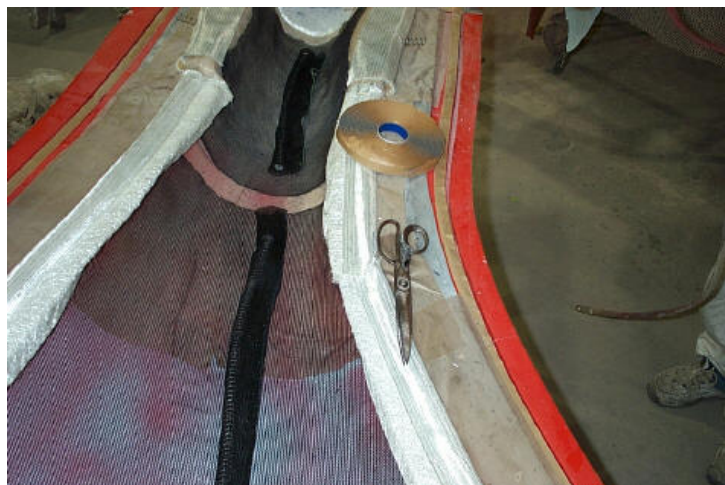
Figure 24 TX-100 Vacuum Bagging (2)
