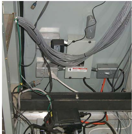
Figure C-2. AC Power Distribution in the Instrument Enclosure.
