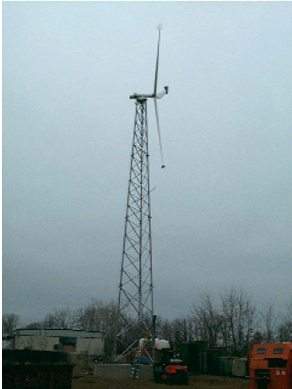
Figure 1.5: Atlantic Orient Corporation's AOC 15/50 turbine installed in Burlington, Vermont. Photograph courtesy of the Atlantic Orient Corporation, www.aocwind.net .
