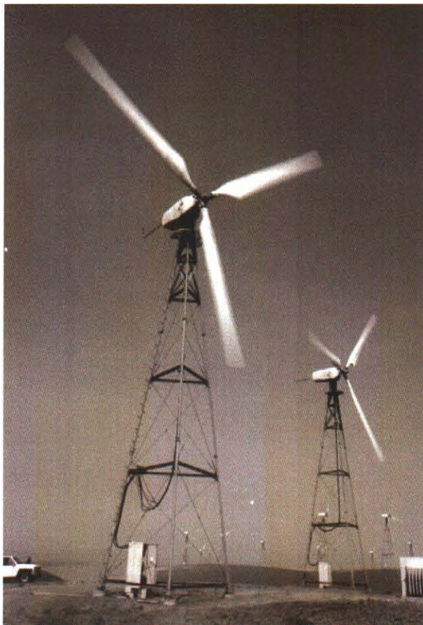
Figure 5. 1 Photograph of the Two Operational Test Turbines
