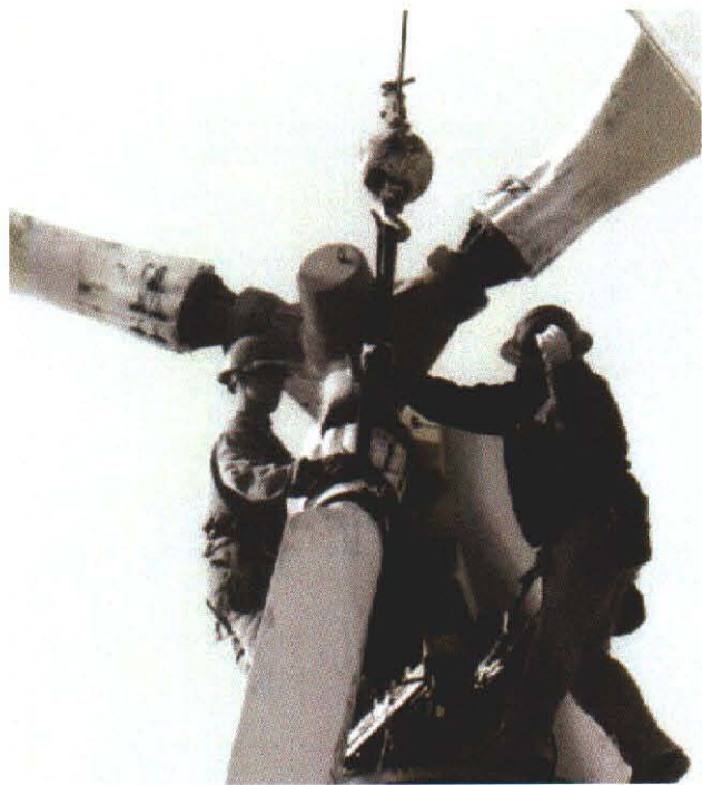
Figure 5.7 Photographs of the Rotor Blade Installation
