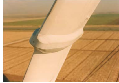
Figure 18. Fairing over Blade-to-Blade Joint.
