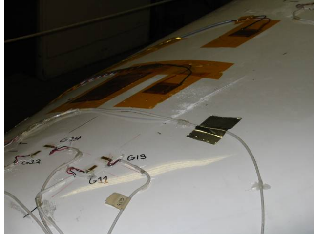
Figure 16: CX-100 low-pressure skin damage area.
