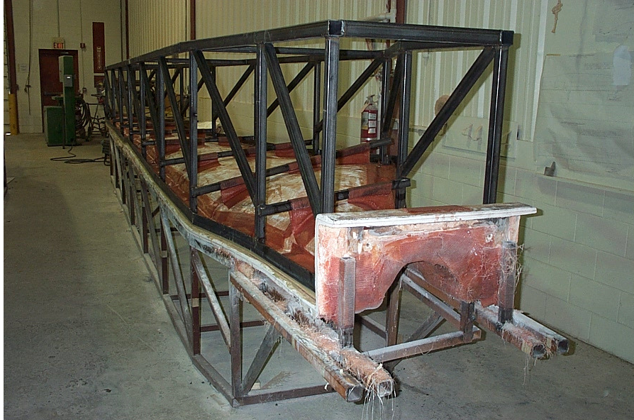
Figure 28 CX-100 Steel Mold Bracing (2)
