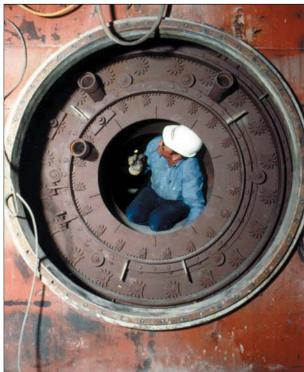
A worker inspects the support ring for the Foster Wheeler low-NO x burner installed in the boiler wall.
