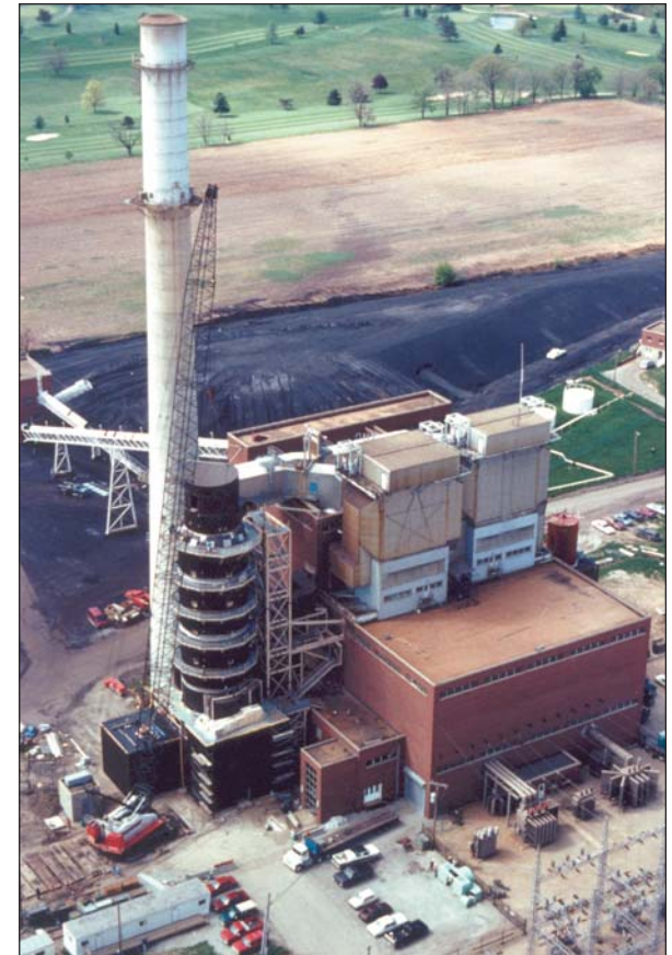
The LIFAC system successfully demonstrated at Whitewater Valley Station Unit No. 2 is being retained by Richmond Power & Light for commercial use with high-sulfur coal. There are 10 full-scale LIFAC units in Canada, China, Finland, Russia, and the United States.
