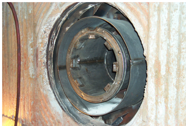
Advanced Low-NO x Burner - 48" Outside Diameter
