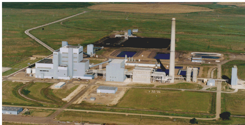
Sunflower's 360 MWe Wall-fired Holcomb Station
