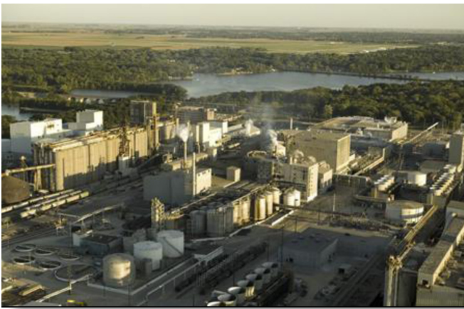
ADM's Agricultural Processing and Biofuels Plant, Decatur, IL.
