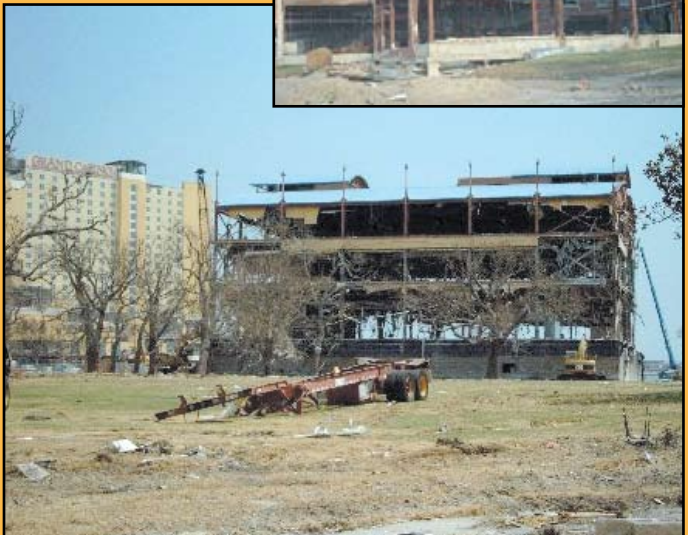
Below: The Grand Casino, in Gulfport, broke into multiple pieces and was relocated by Hurricane Katrina.
