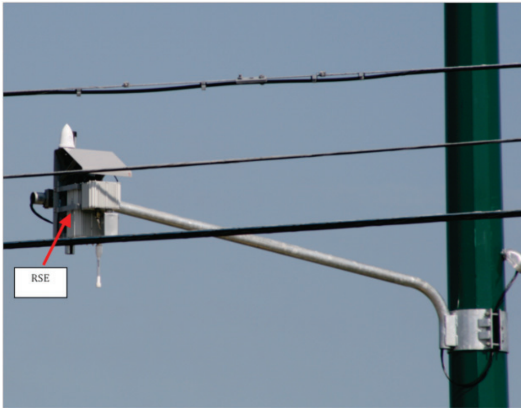
Figure 4-95 Typical RSE Installation
