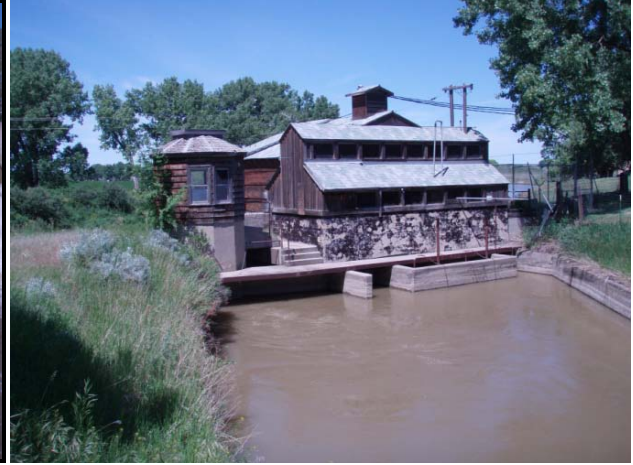
Harlem Irrigation District Pump Station
