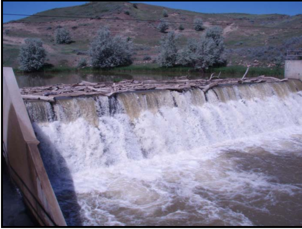
Paradise Valley Irrigation District Diversion Dam
