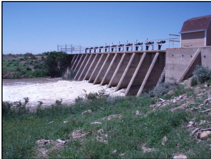
Dodson South Canal Headworks
