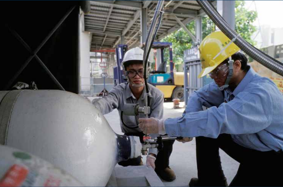
Air Products' facility in Hsinchu, Taiwan. The U.S. company benefitted from help offered by the International Trade Administration's Trade Agreements Compliance Program. (Photo courtesy Air Products)
